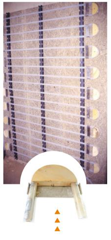
The first bending model for the first system walls was affixed to the pipe on the wall and plastered over
