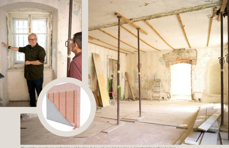
The window reveals are perfect for wall heating, but a well-insulated ceiling is important for surface heating.
