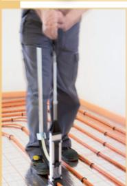
(1) VarioProFile pipe 16x2/Alu0,25 (multi-layer composite pipe).
