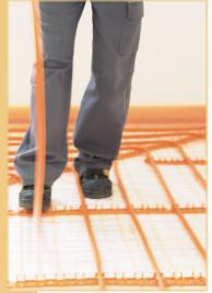
(2) The grid foil (separating layer) is made from 100% polyethylene recycling granulate with a 50 mm graticule and 0.2 mm thickness. One roll contains 50 m<sup>2</sup> of foil. Adhesive tape is used to bond the foil joints. (Roll: length x width = 66 m x 50 mm).
